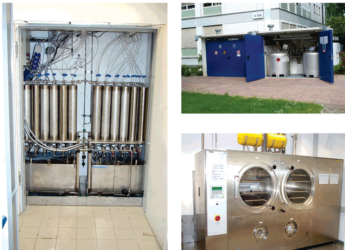
Figure 4. Waste recovery system in unit II, external acetonitrile supply, and waste containers (2 × 1000 L each) and the high capacity freeze-dryer of unit III.
